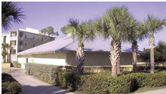
Building Front Photo
