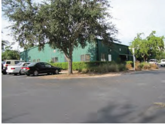
Building Front Photo
