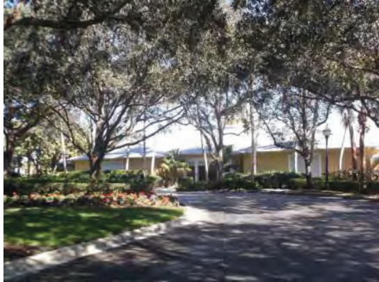
Building Front Photo
