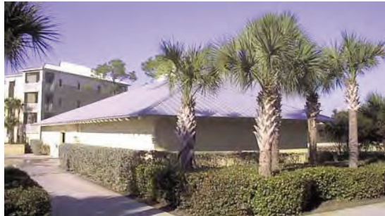
Building Front Photo
