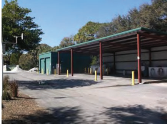
Building Front Photo
