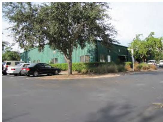
Building Front Photo
